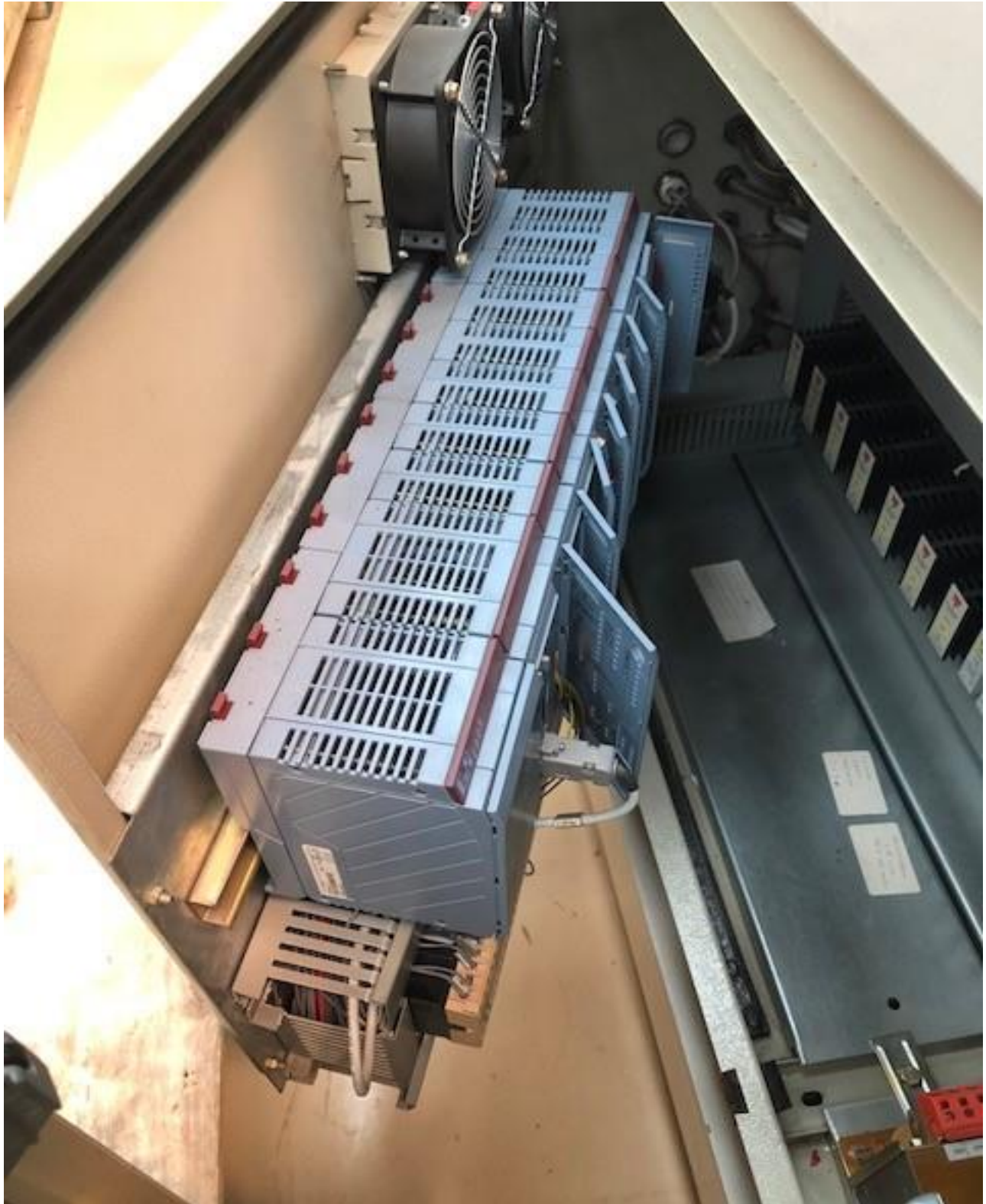
View PLC B&R
