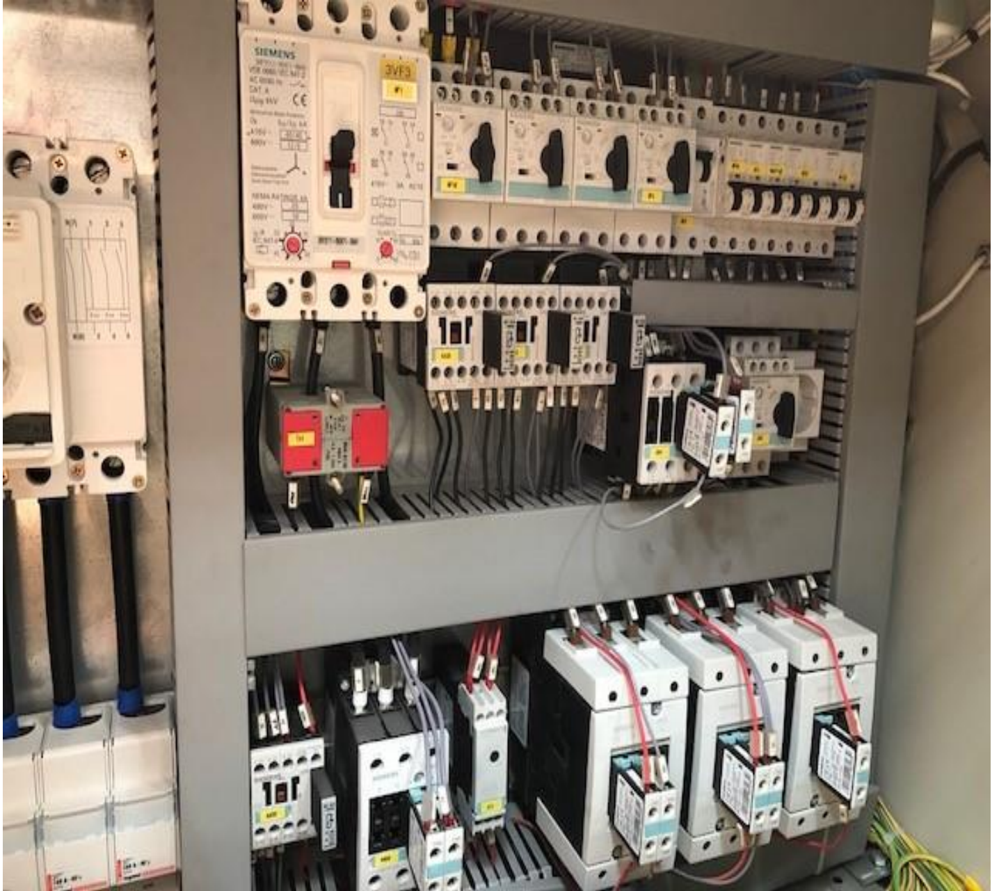
Electric Cabinet Other view
